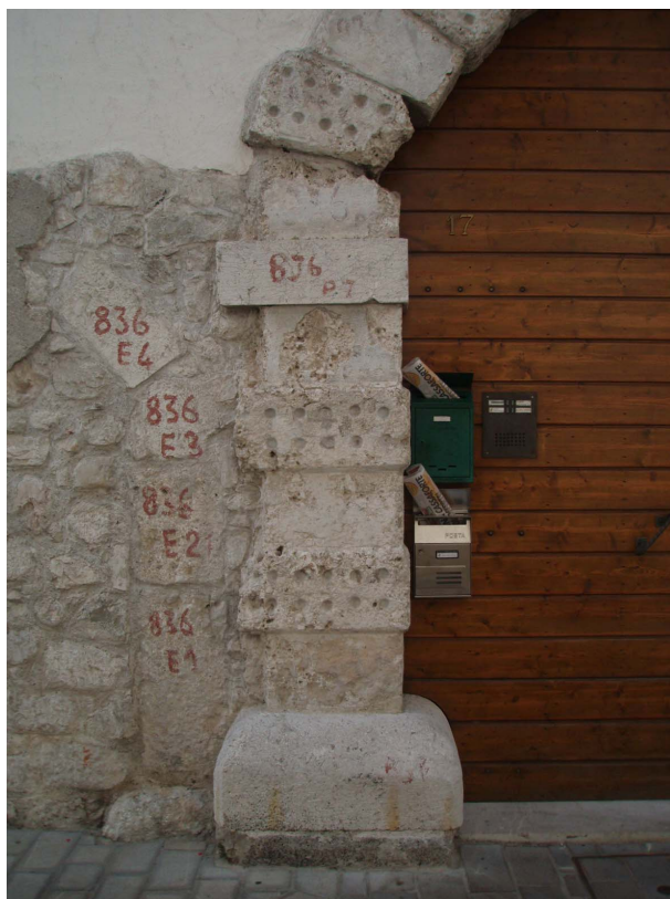
Fig. 3. Markings based on which parts of the buildings were reconstructed after the two earthquakes are still visible on many buildings in the old town of Venzone (photo: Primož Pipan).
