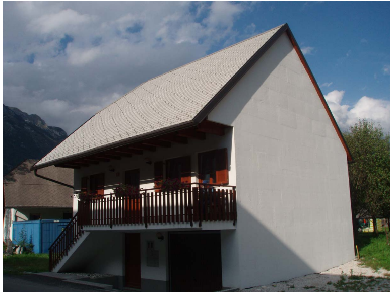
Fig. 9. New house build in Čezsoča after the 2004 earthquake (photo: Primož Pipan).
