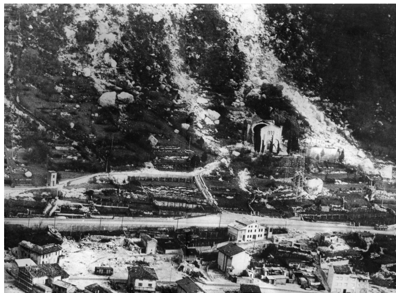
Fig. 4. Portis after the September 1976 earthquake. Rockfalls, which were the main reason for relocating the settlement, can be seen in the background (Archive of Ezio Gollino).
