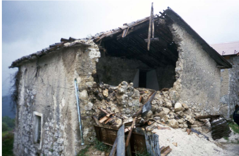
Fig. 7. Damage to buildings in Drežniške Ravne after the 1998 earthquake (photo: Matija Zorn).
