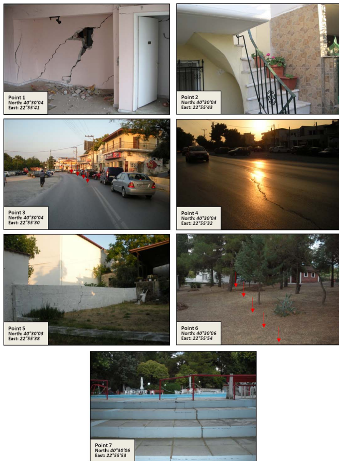
Fig. 11. Field evidences of ground ruptures in Perea. Coordinates are in UTM WGS 84 (projected). Damages witnessed at buildings (points 1 and 2), streets pavement (points 3 and 4), light constructions (points 5 and 7) and natural terrain (point 6).
