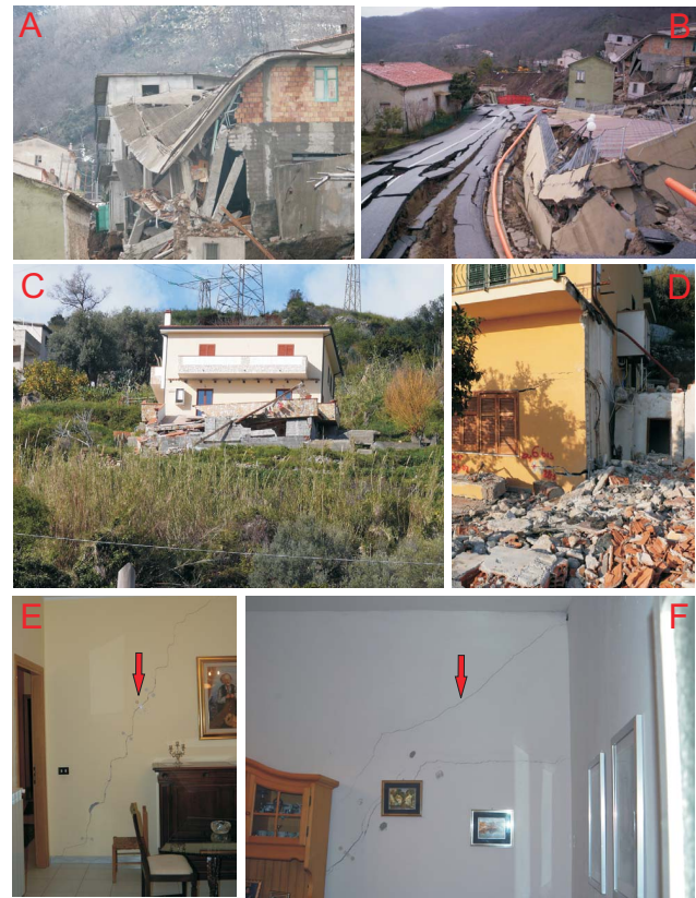
Fig. 5. Some of the effects caused by the analysed mass movements. Photos (A) and (B): case study 1; photos (C) and (D): case study 2; photos (E) and (F): case study 3. The arrows in photos (C) and (D) indicate cracks in one of the damaged houses.
