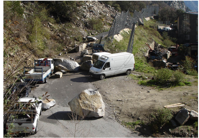
Fig. 4. Individual fallen rock blocks from the rockfall occurred on 20 April 2008.
