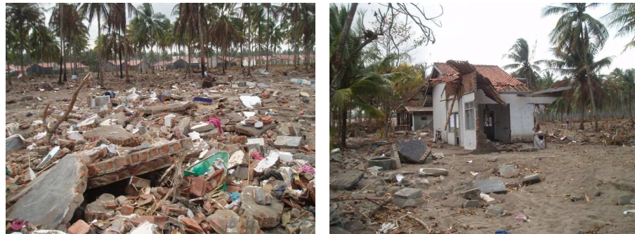
Fig. 12. The remains of traditional brick houses after inundation to a depth of ca. 3 m (a). There were a few partially intact (b).
