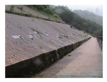
**Fig. 9.** Soil nails installed over a regular grid pattern of boreholes drilled throughout a volcanic saprolite profile.
