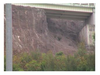
**Fig. 5.** A view from the shotcreted scar of a recent large-volume landslide within a saprolitic profile developed over pyroclastics (Shum Wan Road, Hong Kong). Note the projections of corestones on the nearly vertical surfaces forming the side and rear faces of the scar.
