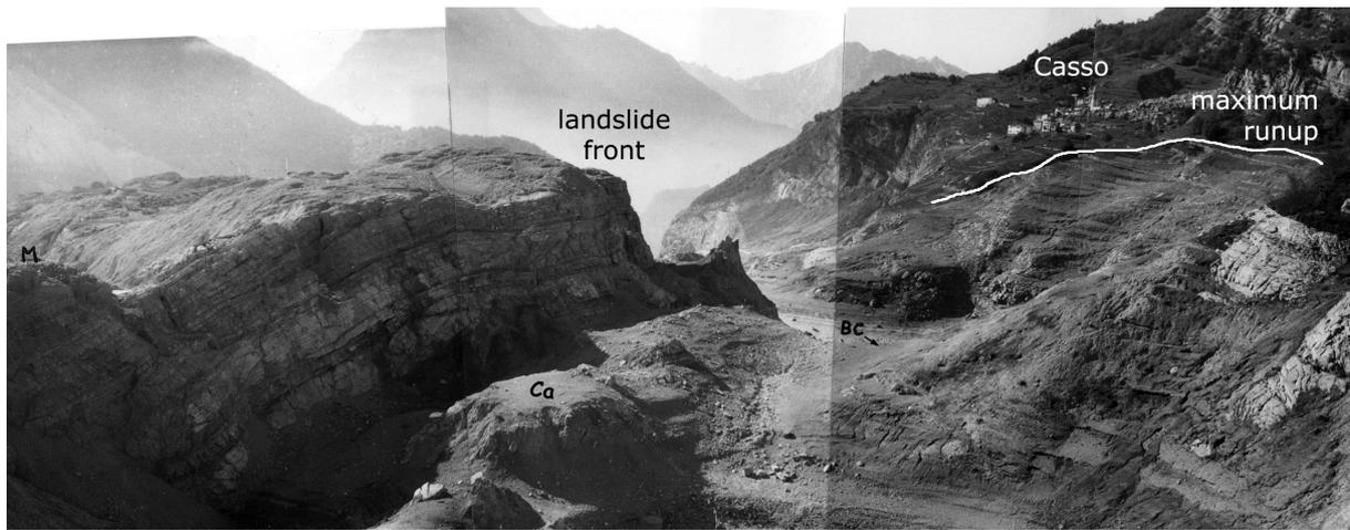
**Fig. 11.** Picture of the Vajont valley after 9 October 1963 landslide. On the right part of the picture the village of Casso is visible, while a white line reports the maximum runup level of the generated impulse wave.
