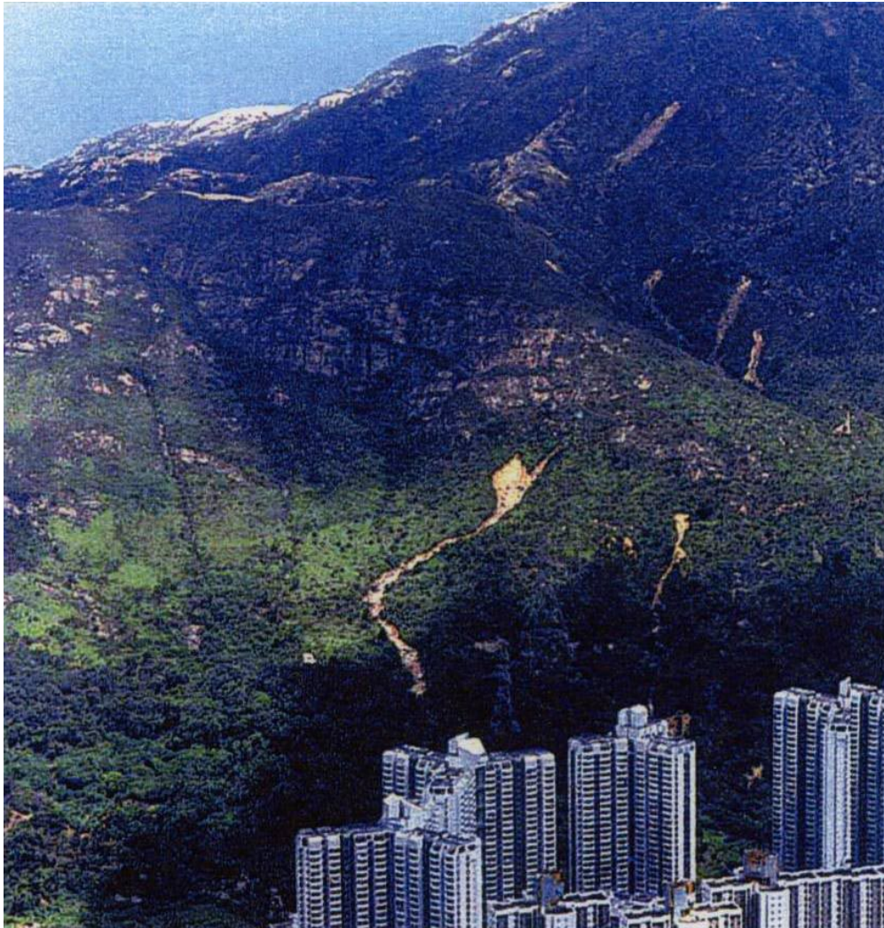
Fig. 1. Debris flows that occurred on 14 April 2000 near Leung King Estate, which is in the foreground.
