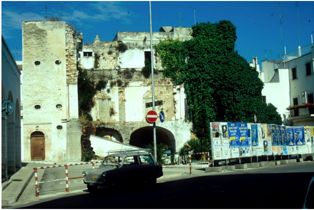
Fig. 10. Buildings involved in cases of subsidence at Largo Porta Grande (photo taken in 1999).
