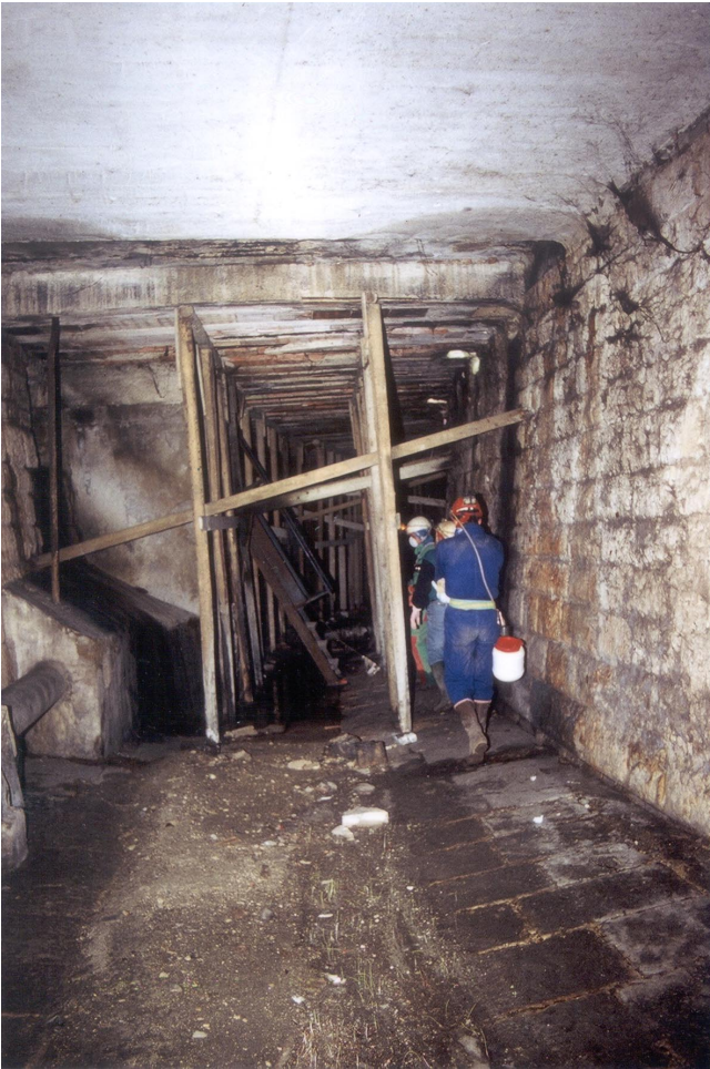
Fig. 13. Inside the Canalone (photo courtesy of Domenico Sgobba).
