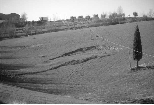
Fig. 5. Another flow with a sliding surface at shallow depth. In spite of their superficial movements, these landslides often produce many damages (in this case an electric line is involved).
