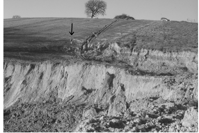
Fig. 7. A detailed view of the main scarp of the Barattano landslide. You can note the man at the top of the scarp (see the arrow) in order to evaluate the real size of the landslide.
