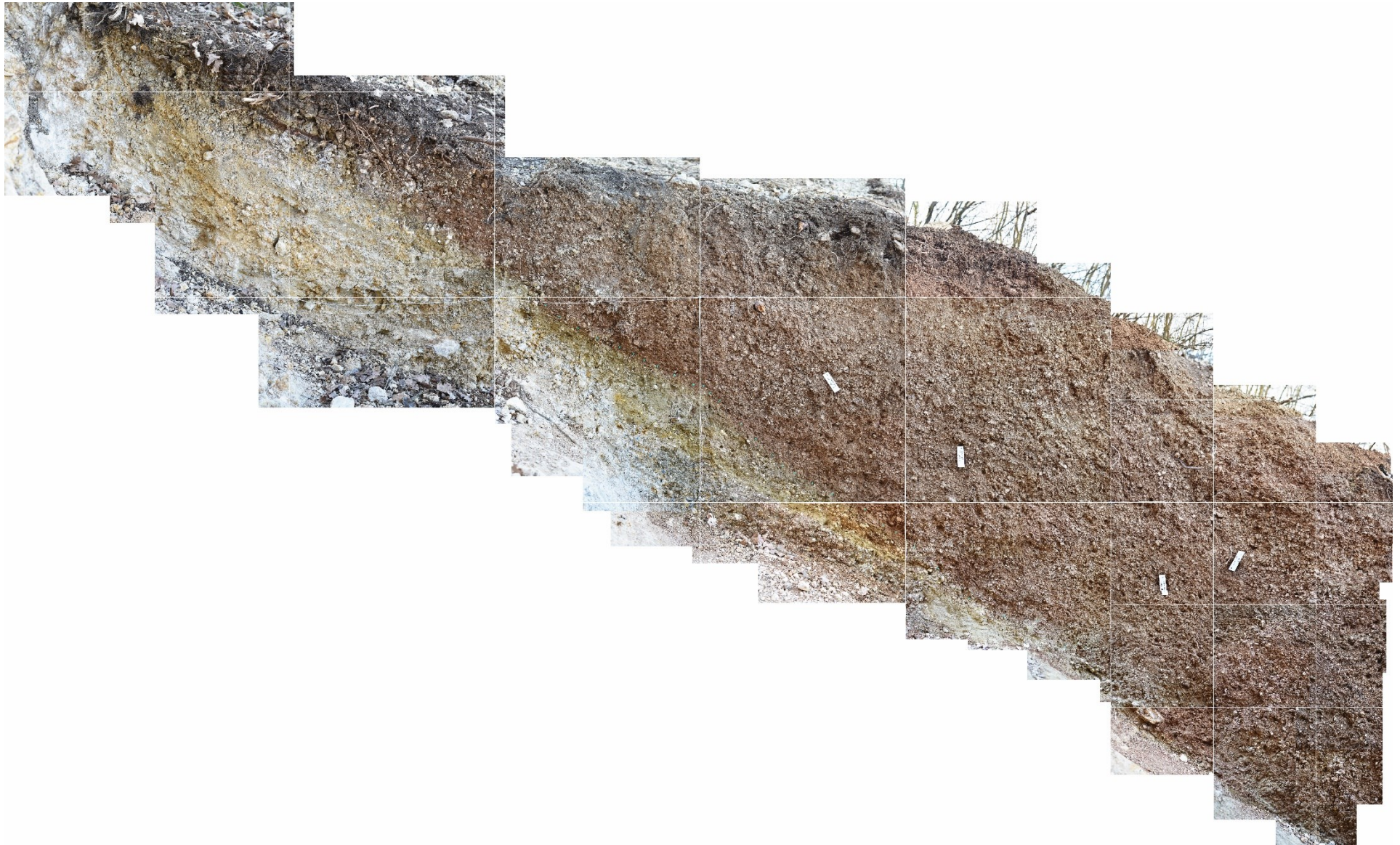
Cantalice T1 South wall
