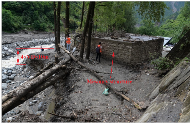
Figure 7. Example informing the determination of the VD threshold. VD in this figure indicates the height difference between the river table and the masonry structure without considering the height of this building.
