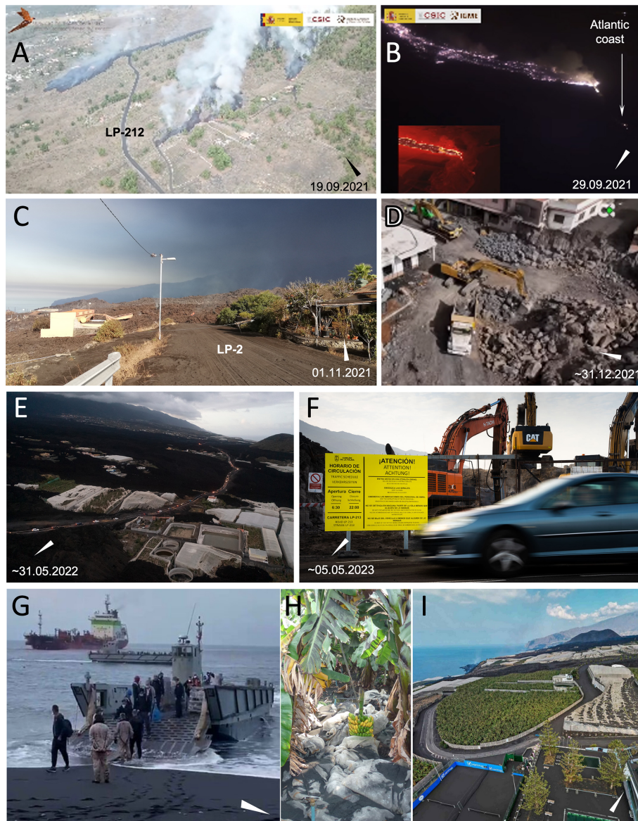
Figure 5. Impacts on critical infrastructure. Arrows indicate the North of the island. (A) Secondary road LP-212 few minutes after the beginning of the eruption on 19 September 2021. UAV flight from IGME (2021a). (B) Lava flows entering into the sea the night of 29 September 2021. UAV flight from IGME (2021b). (C) Primary road LP-2 cut by lava flows and covered by tephra. Telecommunication wood pole damaged (Photo: L. Dominguez). (D) Recovery works start by the end of the eruption (Television Canaria, 2023). (E) New road opening on May 2022 (El Time news, 2022). (F) Time and speed restrictions of the new road (Photo: L. Dominguez). (G) Military boats transporting water and workers from Los Llanos to Puerto Naos (Planeta Canario News, 2021). (H) Water irrigation needs in banana crops (Photo: L. Dominguez). (I) Crops and water tanks South of lava field (Planeta Canario news, 2021).
