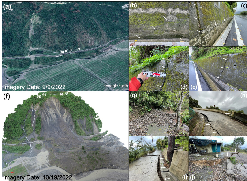
Figure 9. (a) © Google Earth 2022 image before the CL. (b–e) Photos from inspection on 27 May 2022. (f) Drone-based three-dimensional model after the CL. (g–j) Photos of crown cracks of the CL.
