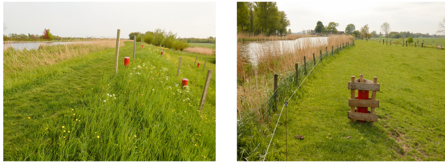
Figure 1. Two examples of canal dikes in the Netherlands: Duifpolder is shown on the left and the Drooggemaakte Geer- en Kleine Blankaardpolder is depicted on the right. In both images, the canal has permanent high water levels close to the crest level (on the left side) and the low-lying polder is mainly used for agriculture (on the right side). The head differences between the canal water levels and water levels in the polders are 2.7 m (Duifpolder) and 4.3 m (Drooggemaakte Geer- en Kleine Blankaardpolder). The red tubes protect the measuring equipment and the piezometers used to measure the hydraulic head. Photos by EURECO/Cyriel Liebrand (2022).
