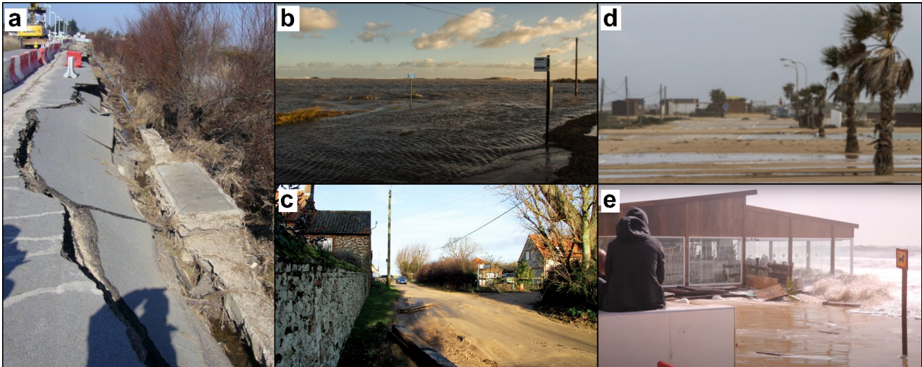
Figure 9. Examples of damage to roads: (a) Route de la Tranche-sur-Mer in the area of La Faute-sur-Mer (France) after the Xynthia event in February 2010; (b) Coast Rd (Salthouse, Holt) and (c) Beach Rd (Holme-next-the-Sea, Hunstanton) in the Norfolk (UK) area after the Xaver event in December 2013; and (d) Carretera Playa de Camposoto in the south of the city of Cádiz (Spain) after the Emma event in March 2018. The images were retrieved from the sources of information collected in the ECFAS database of extreme events and test cases (Souto Ceccon et al., 2021).
