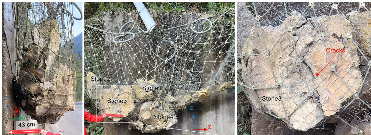
**Figure 4.** Rockfalls piled up in the net.
