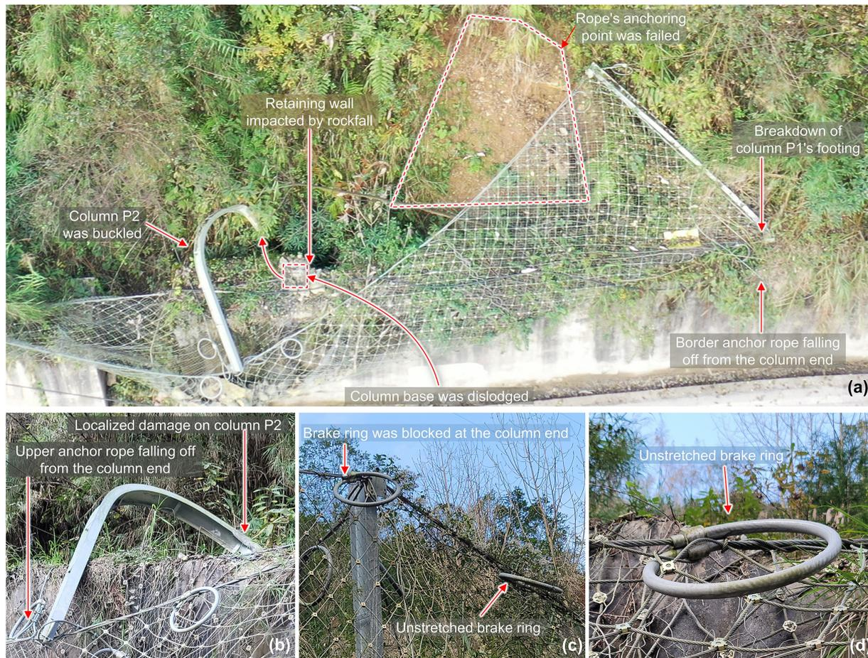
**Figure 6.** Damage phenomena of the flexible barrier. (a) The damaged two-span structure; (b) failure of column P2; (c) non-working brake rings on both sides of column P3 end; (d) connection relationship between the brake ring and the support rope and the steel wire rope net.
