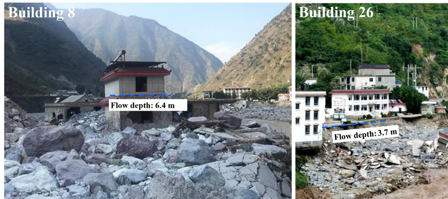
Figure 9. Simulated maximum flow depth of the dam-burst flood at the location of buildings 8 and 6.
