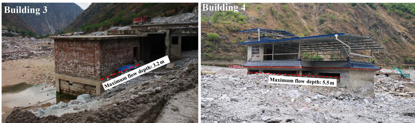
Figure 7. Simulated maximum flow depth of debris flow at the location of buildings 3 and 4.
