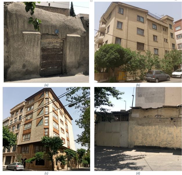
Figure 4. Examples of common residential buildings in Tehran: adobe (a), steel (b), reinforced concrete (c), and masonry (d). Photos by Niloofar Kazemi Asl.
