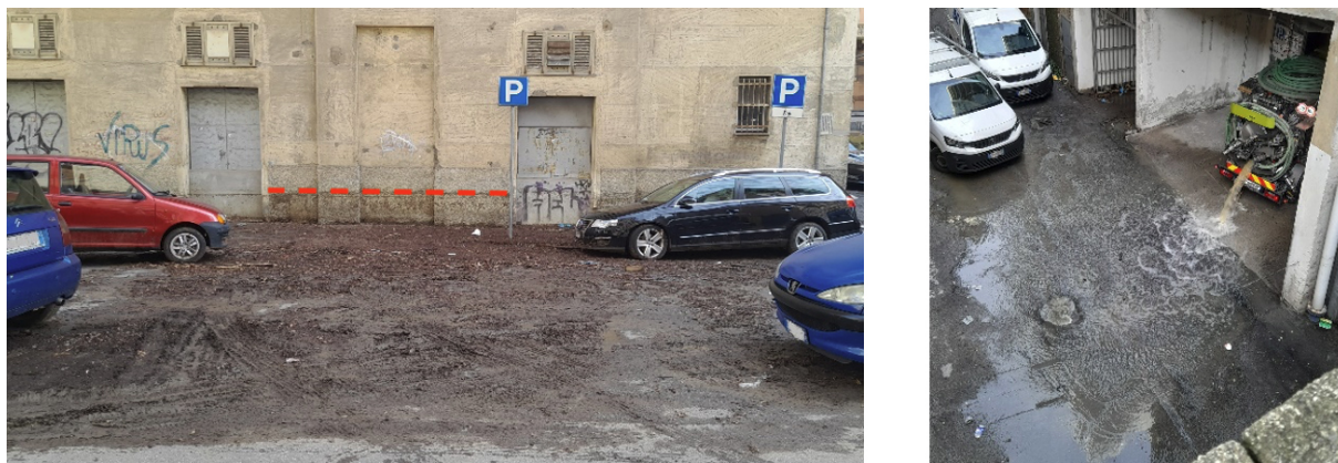
Figure 4. Pictures showing post-event traces of the ground effects of the event analysed. The dashed red line shows traces of the water level reached during the event.
