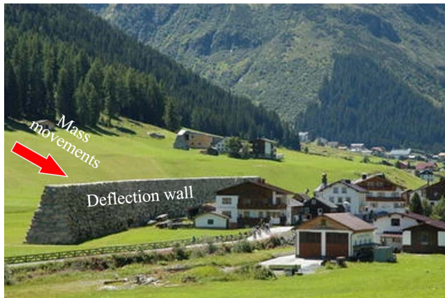
Figure 9. A deflection wall used to protect an entire building ensemble from the impact of medium-magnitude events (Galtur Tschafain, Austria) (Holub et al., 2012).
