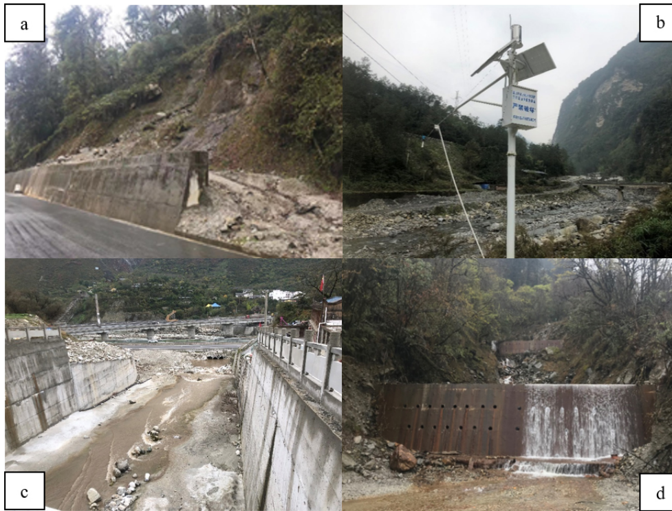
Figure 4. Structural engineering measures to prevent and control: (a) gravity retaining wall, (b) debris flow pre-warning device, (c) discharge chute for debris flow, (d) permeable type of retaining dam for debris flow.
