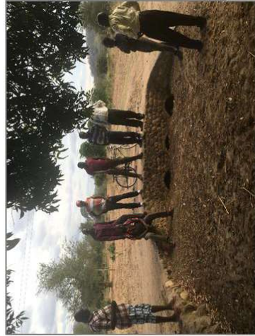
Nkomi river culvert built in 2005, filled by sands. (20/11/2018).
