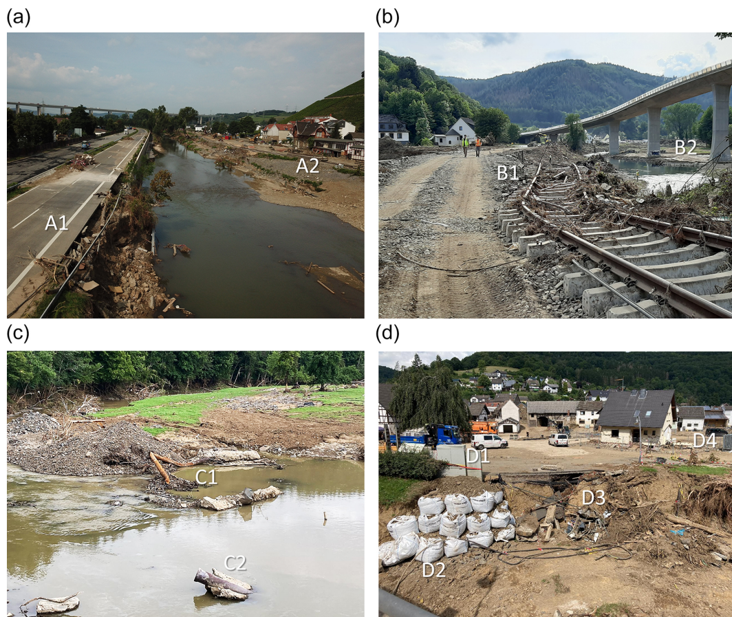
Figure 1. Damage in the Ahr valley, Germany (images taken on 11 August 2021). (a) Destruction of federal highway B266 (A1) and railway (A2) near Heimersheim. (b) Further upstream in the Ahr valley (Altenburg), large stretches of the Ahrtalbahn railway have been destroyed (B1) and the few remaining road and rail bridges show signs of temporary repairs (B2). (c) Riverbed erosion uncovered and destroyed many cables supposed to lie more than 80 cm below surface level (C1) as well as sewers (C2). (d) Inundated electricity distribution infrastructure (D1), road erosion and stabilization (D2), uncovered cables (D3), and collapsed buildings in Schuld. Pictures by Margreet van Marle/Deltares/GEERassociation, distributed under Creative Commons Attribution 4.0 license.
