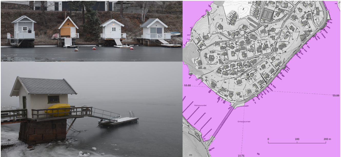
Figure 2. Buildings on piers or pillars above the water surface, like here at Ormøya close to Oslo, are erroneously mapped as flooded for present MHW (violet). Photo: Kristian Breili. Map data shown are provided by Geonorge and Norway Digital consortium and subject to the Norwegian License for Open Government Data (NLOD) 2.0 and Creative Commons BY 4.0 (CC BY 4.0).
