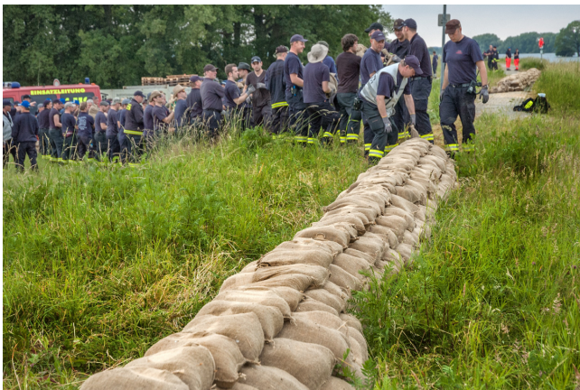
Figure 2. Firefighters during the Elbe flood in 2013, setting up a sandbag dam to raise a dike.
