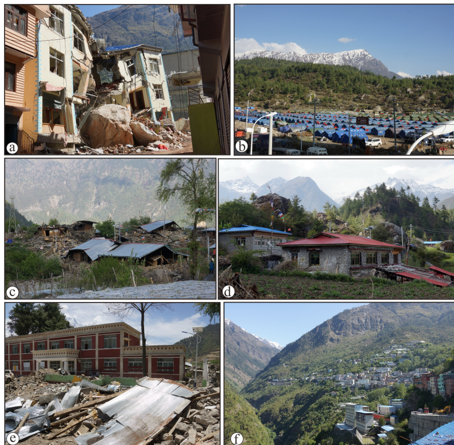
Figure 4. Typical earthquake damage in southern Tibet and comparison of houses of different construction (locations shown in Fig. 5). (a) Huge rockfall that smashed the resident committee office building at Disigang Village, about 0.7 km south of Zhangmu, where seven persons were killed (intensity IX) (site 1, Fig. 5a). (b) A temporary settlement for earthquake survivors at Jilong. (c) Destroyed houses of stone block masonry or adobe construction in Jifu Village southwest of Jilong (intensity VIII) (site 8, Fig. 5b). (d) Houses of cement-bonded stone or brick construction in Jifu Village (intensity IX). (e) Destroyed old houses and new buildings that are still standing at Sale Town Primary School (intensity VIII) (site 7, Fig. 5b). (f) Few collapsed houses at Zhangmu due to the brick structure or reinforced concrete construction (intensity IX).
