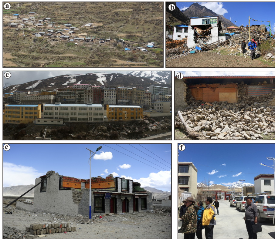
Figure 3. Building damage resulting from different earthquake intensities. (a) Many of the old stone pile or mud brick houses collapsed, but the new brick houses rarely collapsed at Gangba Village in Sale Town in the intensity VIII zone. (b) Similar building damage at Zhuobude Village of Rongxia Town in the intensity VIII zone. (c) Most buildings with a brick or concrete structure did not collapse, but many walls showed obvious damage at Nyalam City located in the intensity VIII zone. (d) Some walls of the stone pile or mud brick houses collapsed at Rema Village, Jilong County, in the intensity VII zone. (e) Similar building damage at Chentang Town, Dinggyê County, in the intensity VII zone. (f) Most of the houses remain intact, and only few or individual walls of buildings had apparent small cracks in Gyirong City in the intensity VI zone.
