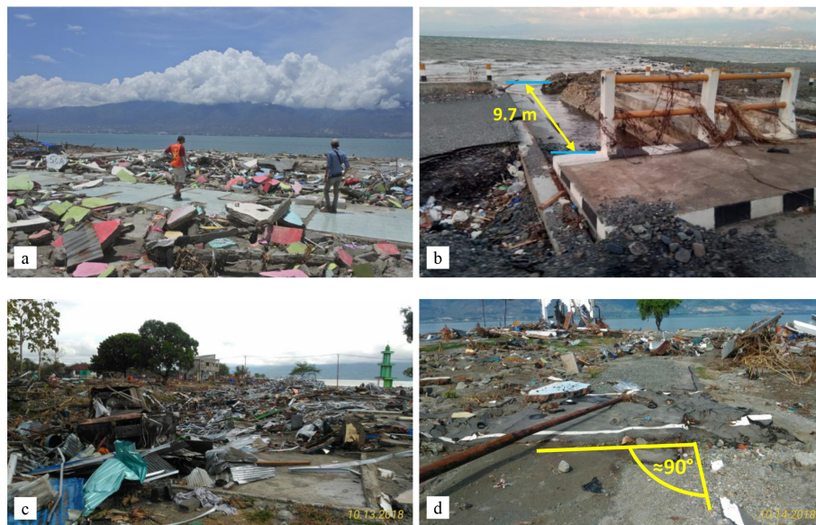
Figure 6. (a) Damage caused by the tsunami in Tondo, a residential complex where a lot of private boarding houses were inhabited by students at the University of Tadulako, (b) a reinforced concrete bridge on Cumi-cumi Road in Palu City was shifted by 9.7 m by the tsunami, (c) Mamboro Village with 90 % of houses destroyed, and (d) asphalt layer of small road turned 90° in Tondo.
