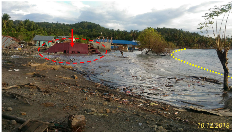
Figure 12. Quick land subsidence in Lero Village. Photograph taken 2 weeks after the event. Some houses dropped suddenly, around 3–4 m, when the earthquake occurred. Residents of these houses, especially those indicated by the oval, could not evacuate in time. The yellow dotted line is the former coastline.
