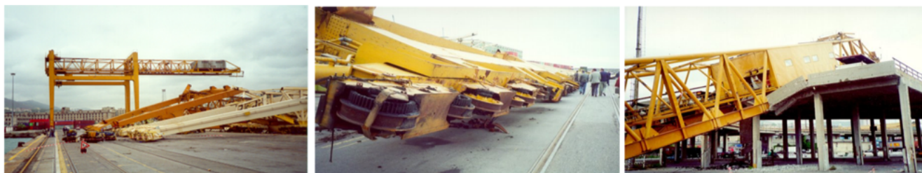
Figure 3. Damages caused by the thunderstorm downburst that occurred in the port of Genoa (Italy) on 31 August 1994 (Photos by the Authors).
