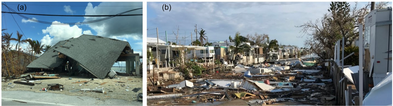
Figure 2. Photos of damage in (a) Big Pine Key: storm surge damage beside a waterway (left side of building) and (b) Marathon: trailer community with house debris filling a waterway.
