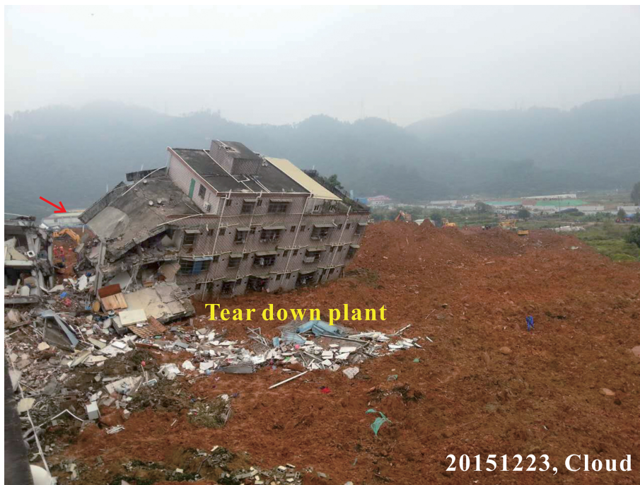
Figure 15. The damage of buildings in the industrial park.
