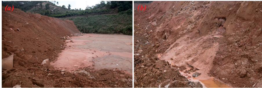
Figure 16. Evidence of liquefaction near the opening of the failed slope.
