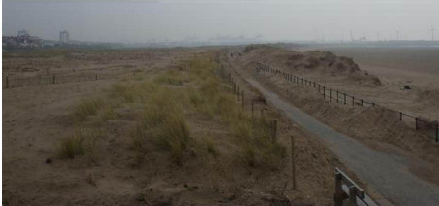
Figure 1. An example of a UK site (Crosby, North West England) where the dune system has built up around an engineered defence (the pathway runs along the top of a seawall and revetment) due to its position relative to the spring high-tide level, thereby changing the management issues in this location from flood risk to safe access.
