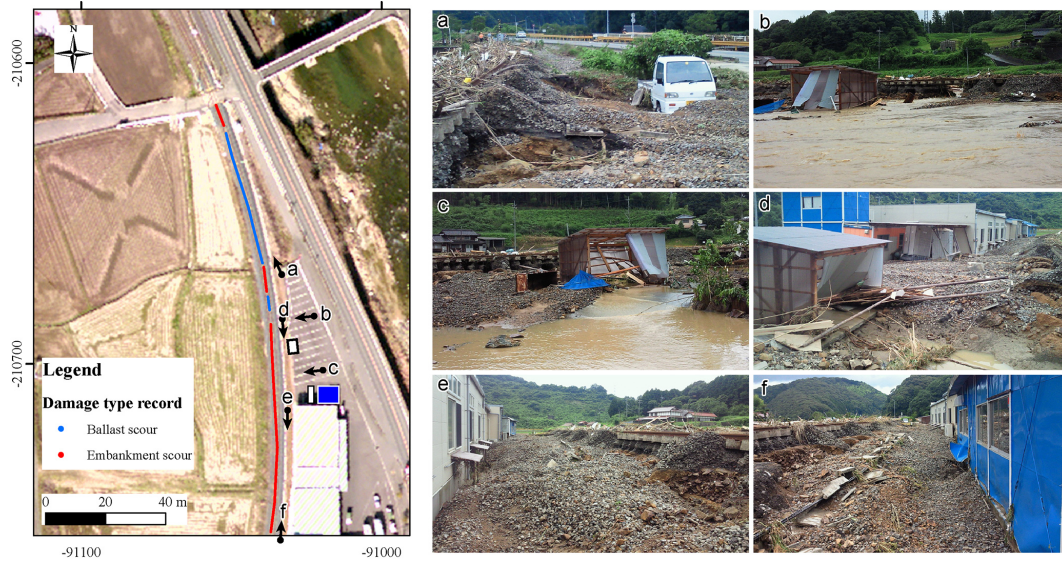
Figure 7. Example of the photos showing the status of the railway ballast–embankment scour just after the flood. Shooting location and direction of each photo are both plotted in the left orthorectified aerial photo taken in February 2012 (photo source: M. Kikunaga).
