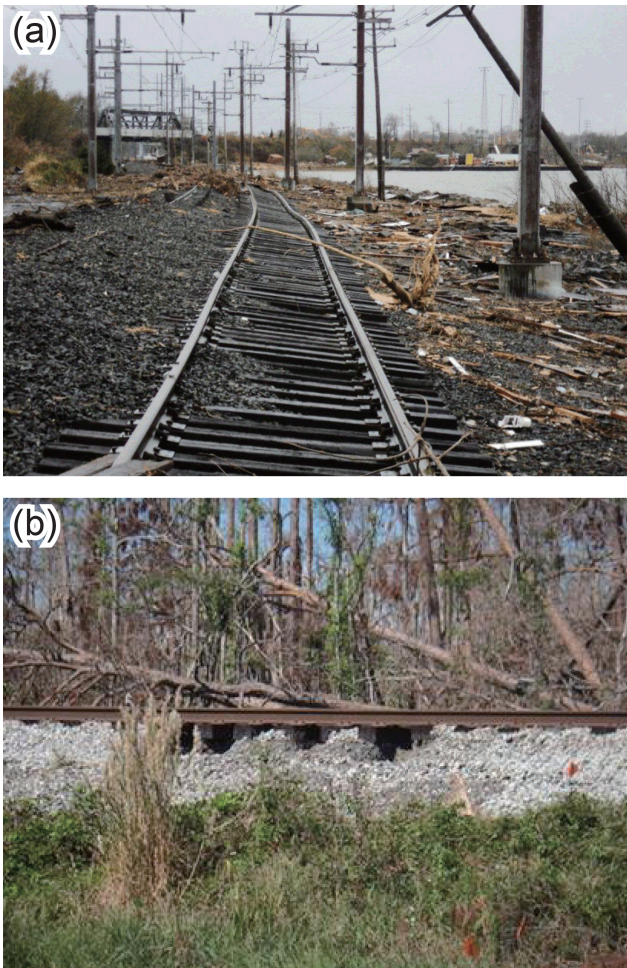
Figure 1. Railway ballast scour failures: (a) New Jersey Transit tracks in New Jersey, USA, after Hurricane Sandy in 2012; (b) CSX railroad tracks in Mississippi, USA, after Hurricane Katrina in 2005 (photo credits: New Jersey Transit, a).
