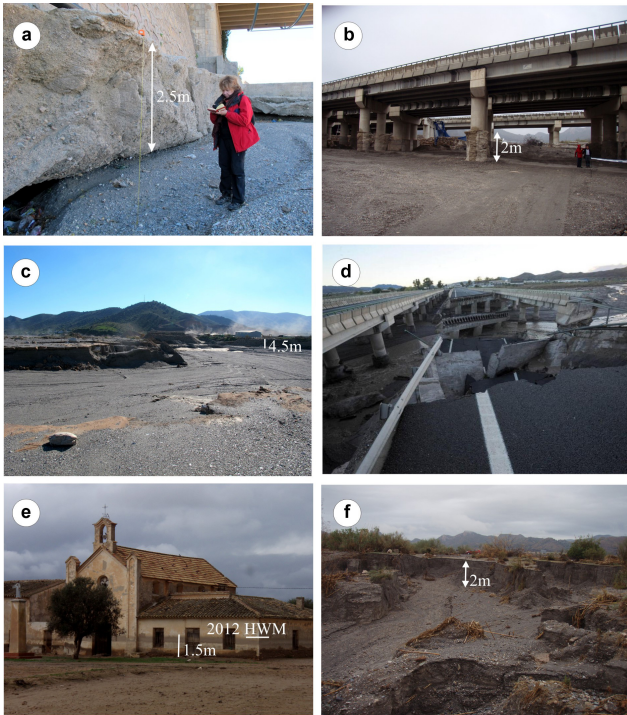
Figure 6. Pictures from the 2012 flood effects. (a) Entrenchment of 2.5 m below Puerto Lumbreras Bridge. (b) In-channel gravel quarry in Nogalte fan apex showing 4.5 m channel entrenchment. (c) Escucha Chapel in Nogalte distal fan area showing the 1.5 m high water mark from 2012 event. (d) and (e) Gravel mining impact on A-7 highway bridge after 2012 event; pillars are exposed in 2 m. (f) Headwards erosion due to gravel mining in the B ejar Rambla.
