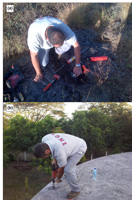
Figure A2. Installation of (a) Lacayo benchmark (LACA) on rocky lava outcrop and (b) Tanque benchmark (TANQ) on existing reinforced concrete structure.
