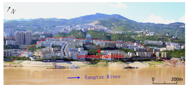
Figure 3. The residential buildings on the Sanmashan landslide in the new Fengjie town after the Three Gorges Reservoir filled with water (photograph taken 6 July 2013). The elevation of the Yangtze river water level is about 147 m a.s.l.
