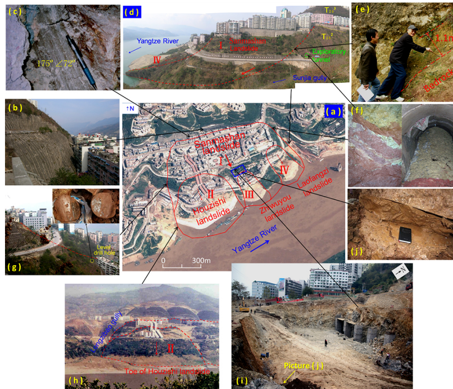
Figure 14. Various views of the Sanmashan landslide. (a) Quickbird image map (September 2004). Area is subdivided into four domains (I–IV). (b) The crown and scarp of the Sanmashan landslide. (c) Slickenside discovered in a foundation excavation in 2000 (taken by Zhengquan Cui). (d) Landslide seen from the east. (e) Sliding zone near the eastern boundary. (f) The sliding zone in the exploratory tunnel. (g) The sliding scarp in a horizontal drilling hole near the western boundary. (h) The western slide boundary and the toe of the Houzishi secondary landslide in 2000. (i) Large foundation pit (in 2013), in which the sliding zone of the Zhiwuyou secondary landslide is exposed (see also (j) and Fig. 15).
