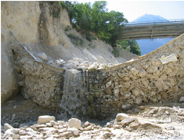
Figure 1. Filled debris-flow barrier in the Illgraben, Switzerland (Wendeler, 2008).
