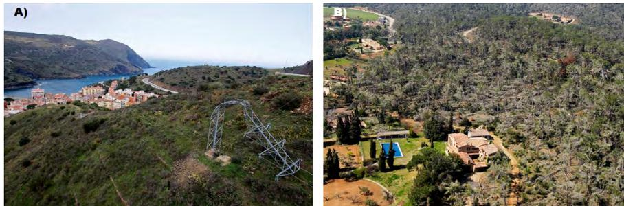
**Fig. 4.** (a) High-voltage power-transmission tower destroyed near France (Port-Bou) by wind and the weight of the wet snow. Source: [www.elperiodico.com](http://www.elperiodico.com). (b) Fallen trees due to the effect of snowfall and wind (Les Gavarres, Girona). Source: [www.elperiodico.com](http://www.elperiodico.com).
