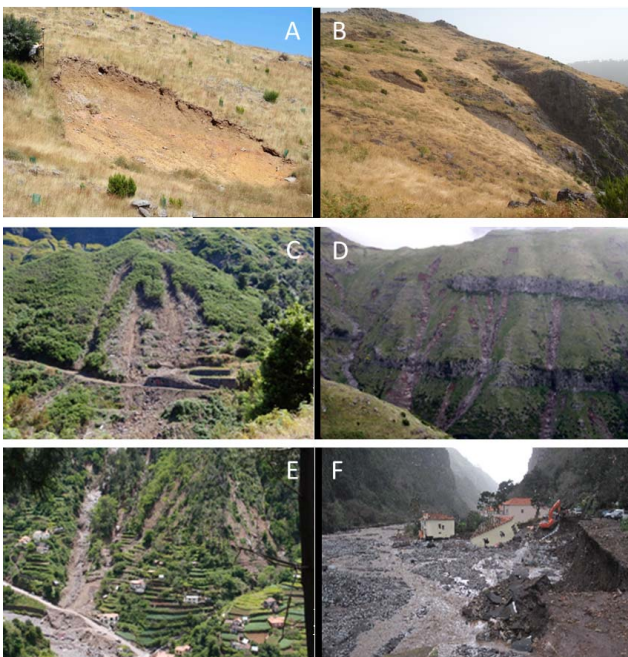
Fig. 2. Shallow landslides triggered during the 2010 event: (A) and (B) – soil-slips; (C), (D), and (E) – soil slip-debris flows; (F) – material damages.
