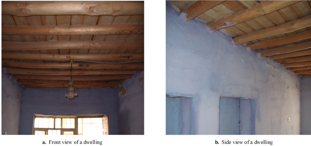
Fig. 11. Views from the interior of the traditional roof system with wooden sheathing.
