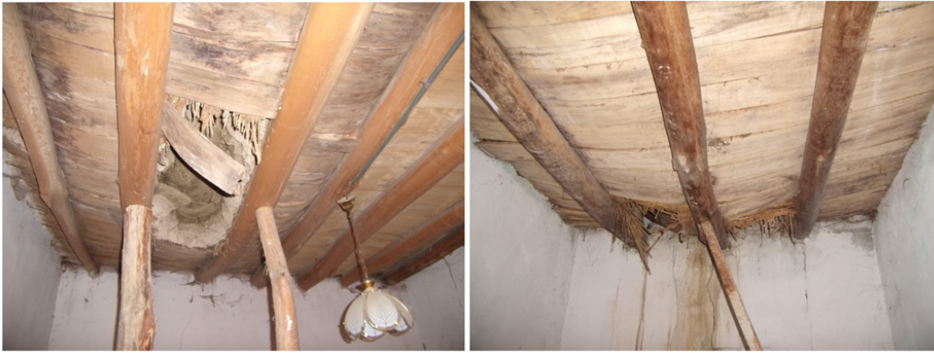
Fig. 21. Partially damages observed in a heavy flat roof system.
