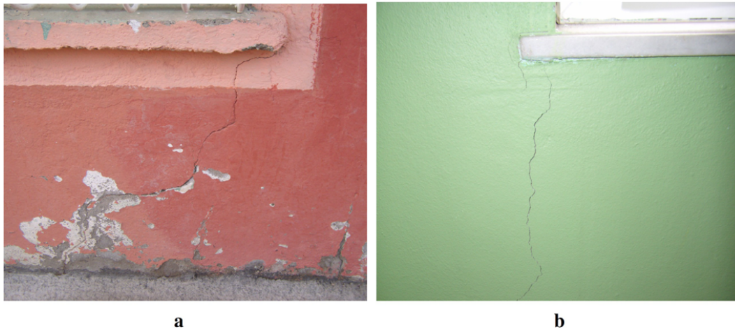
Fig. 27. Slight cracks at sill parts of window openings.
