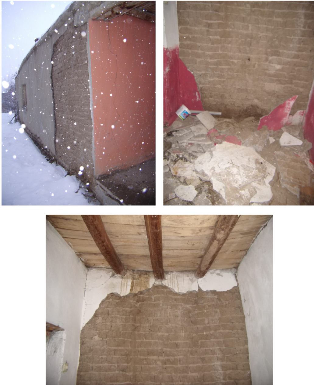
Fig. 19. The exterior and the interior plaster spalling at the adobe walls.
