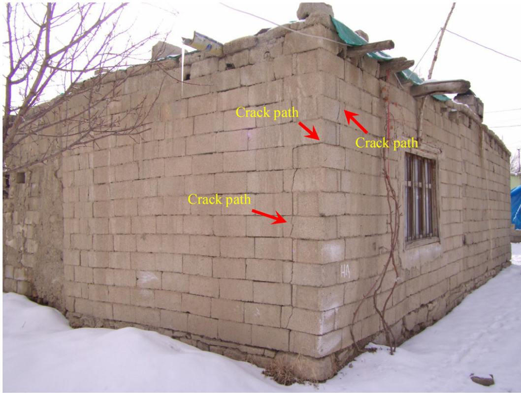
Fig. 23. Crack propagated from one wall to the other in perpendicular direction at the building corner.
