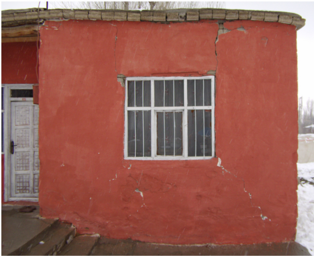
Fig. 16. The cracks developed at the sill and spandrel parts of a masonry wall with a window opening.
