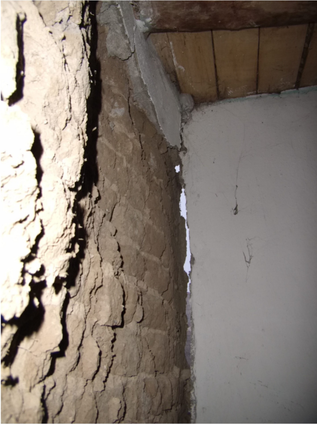
Fig. 20. The interior plaster spalling and severe separation that occurred in the intersection of the walls in an adobe building.
