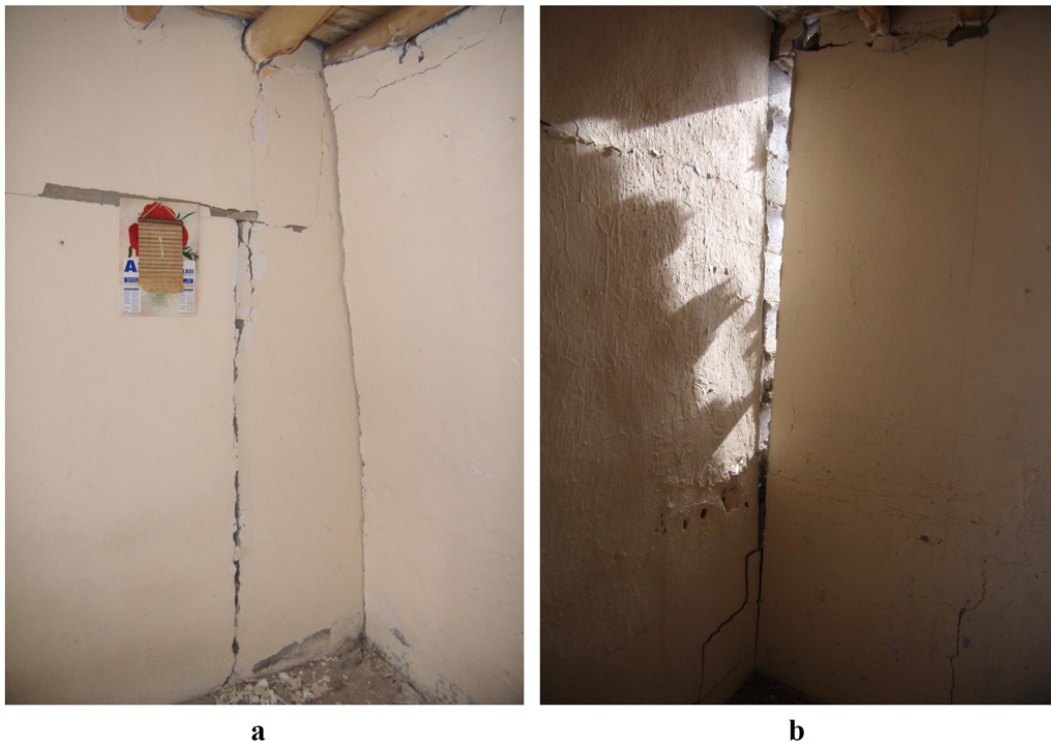
Fig. 14. Severe damages due to overturning moments and developed gaps at the intersections of the bearing walls.
