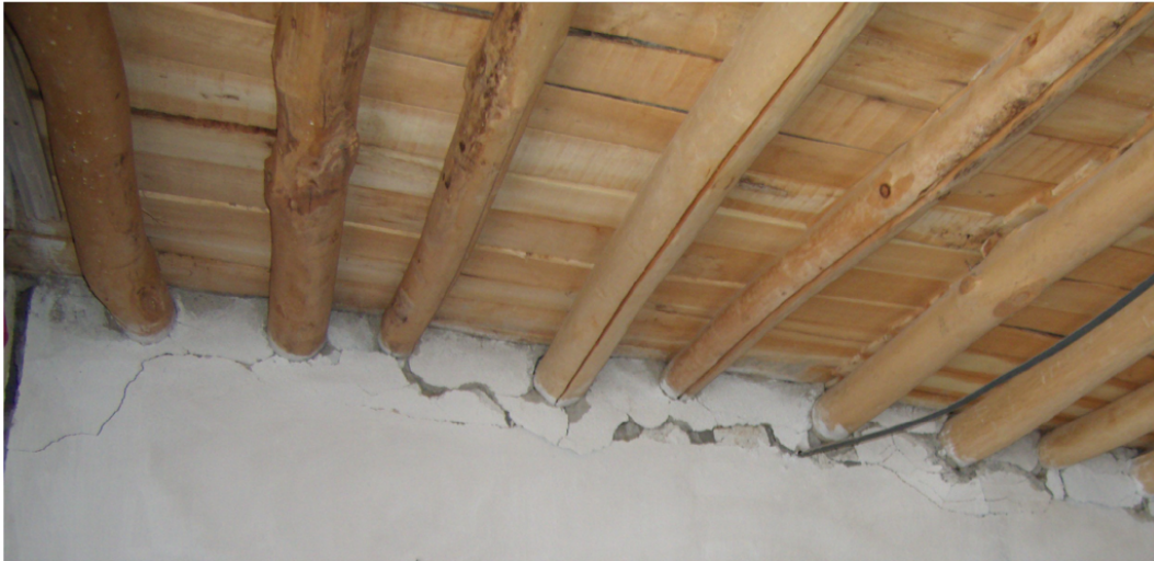
Fig. 18. The plaster spalling under the log ends and longitudinal cracks in some logs.
