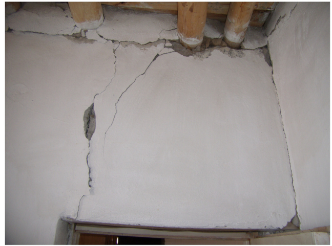
Fig. 17. Plaster spalling and the cracks developed at the spandrel part of a masonry wall above the door opening.
