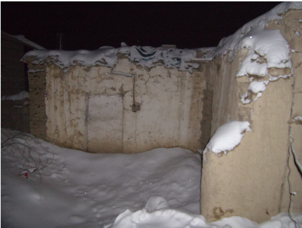
Fig. 22. A partially collapsed adobe building where the debris was removed.
