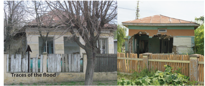
Fig. 2. Example of damaged houses in Vadu Roșca after the flood of July 2005 (pictures: F. Salit, June 2012).
