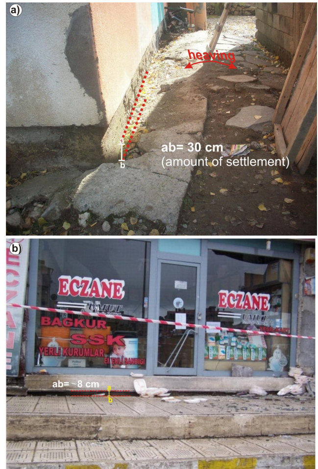
Fig. 12. (a) Liquefaction-related settlement that occurred under a house at Çelebibağı, Erçiş and (b) liquefaction-related settlement at the mid-part of the Erçiş Basin (CGE, 2011).
