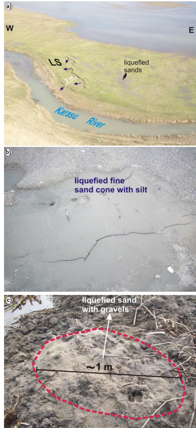
Fig. 10. (a) Sand boils and ejection of liquefied soils into the surface through a ground crack in Karasu Delta, (b) sand cone of liquefied fine-grained soil in the eastern shores of Lake Van around Çitören village, and (c) sand boil of liquefied sand with gravels in the northern shores of Lake Van around south of Çelebibağı.
