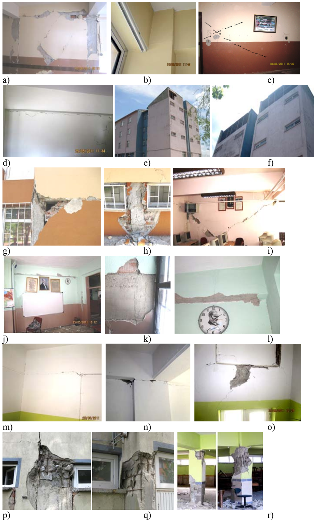
Fig. 5. Observed typical damages at investigated buildings.
