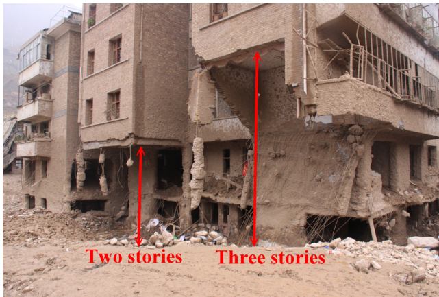
Fig. 5. Differing extent of damage to building H by longitudinally decreasing impact force.
