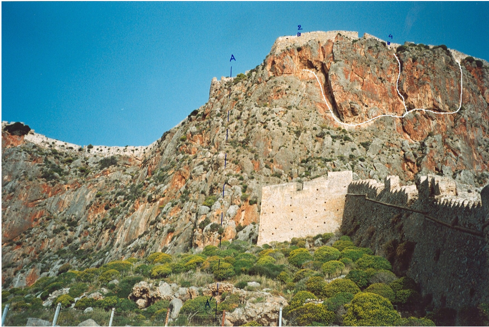
Fig. 10. Photo of a section of the slope having hanging blocks with very large dimensions.
