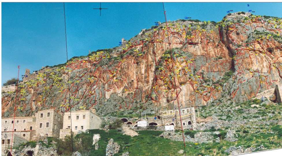
Fig. 5. Potentially unstable blocks in area 4 and 5 are shown in yellow.
