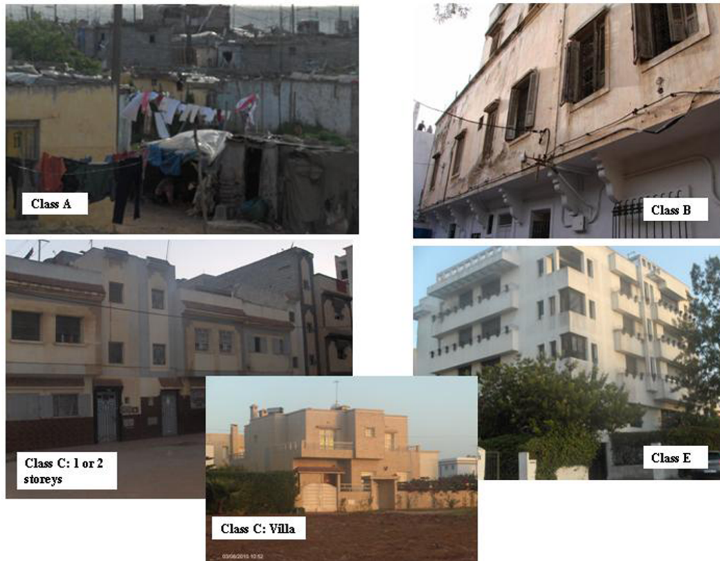
Fig. 4. Examples of constructions of Rabat and Salé representing various classes of building vulnerability.
