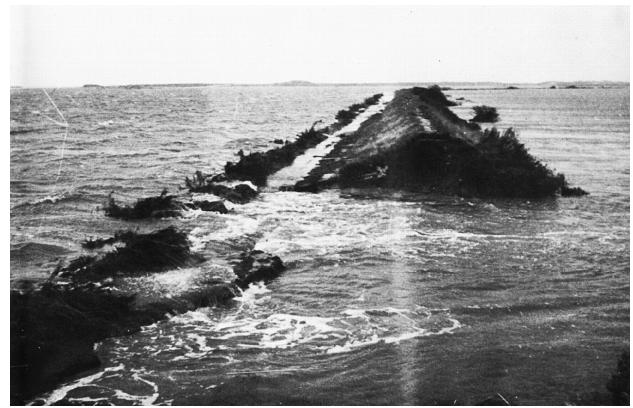
Fig. 2. Typical breach in the flood defences during the 1953 floods.
