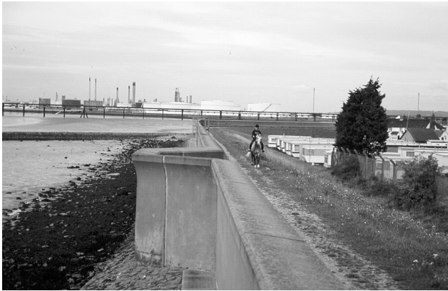
Fig. 10. Improved flood defences built to protect Canvey Island following the 1953 flood.
