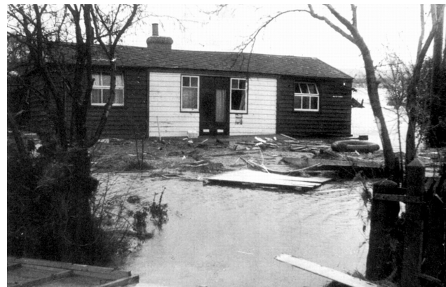
Fig. 6. A typical wooden house that was swept away in the 1953 flood.
