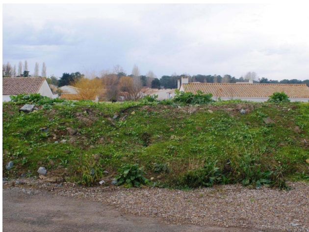
Fig. 7. Single storey houses located behind coastal flood defences in La Faute-sur-Mer.
