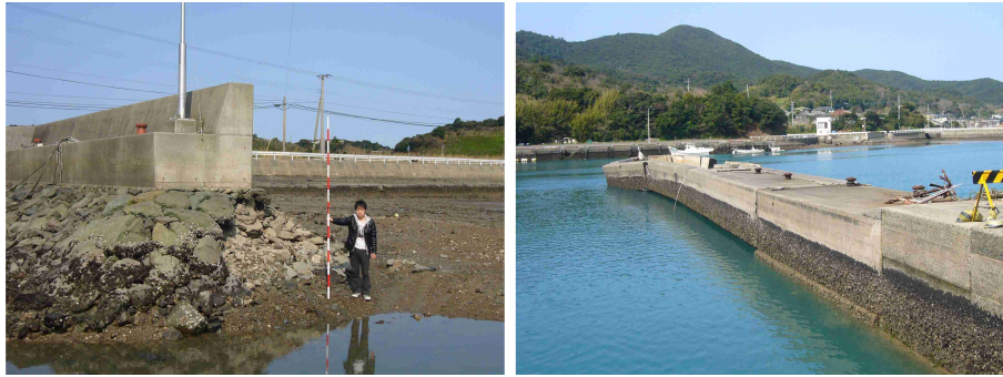
Fig. 4. Photographs of dike damage at Urauchi Bay, Kamikoshiki Island, provided by T. Asano, Kagoshima University.
