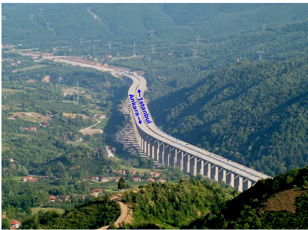
Fig. 2. General view of the Bolu Viaduct (modified from www.bolu.net , 2010).
